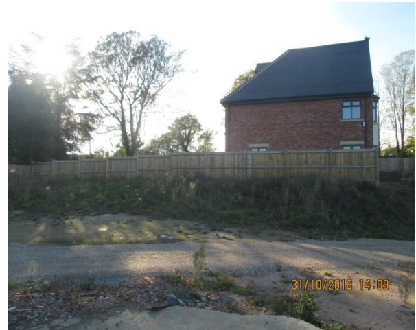
East elevation of no. 7A Middleton Crescent
